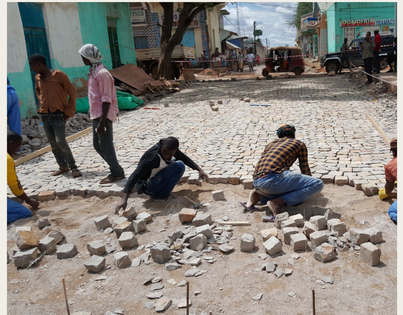
Cobble stone work in progress in Baidoa, Somalia
