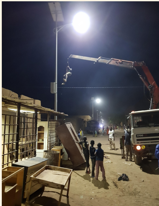
Solar streetlight installation, Gao.
