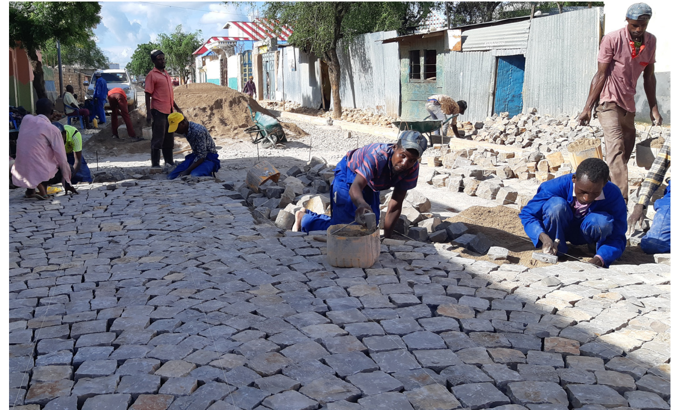
Baidoa Cobble Stone Road Project, Somalia
