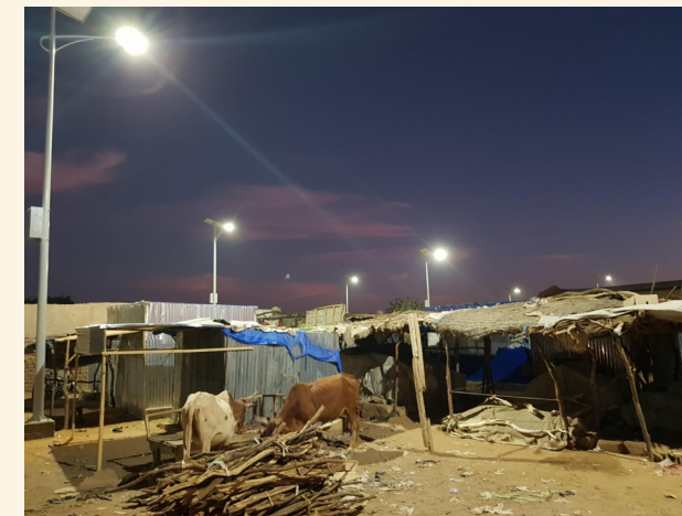
Photo: NIS. Solar streetlights at a market in Gao, Mali
