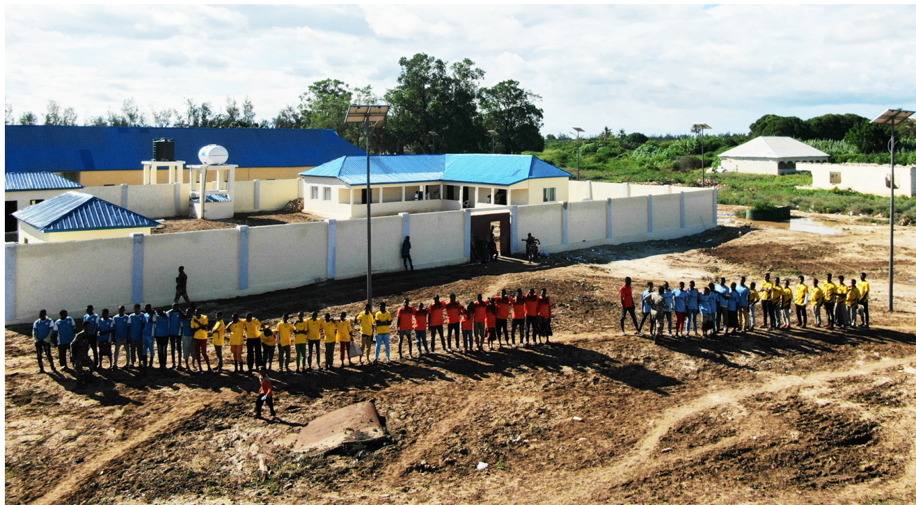
Construction of Awdhegle Primary School, Somalia
