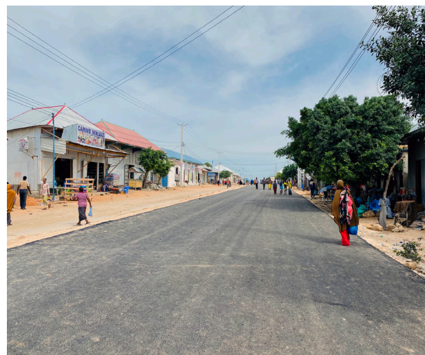
Dayniile Road Construction, Somalia
