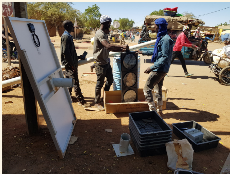
Photo: NIS. Solar streetlights installation team in Gao, Mali
