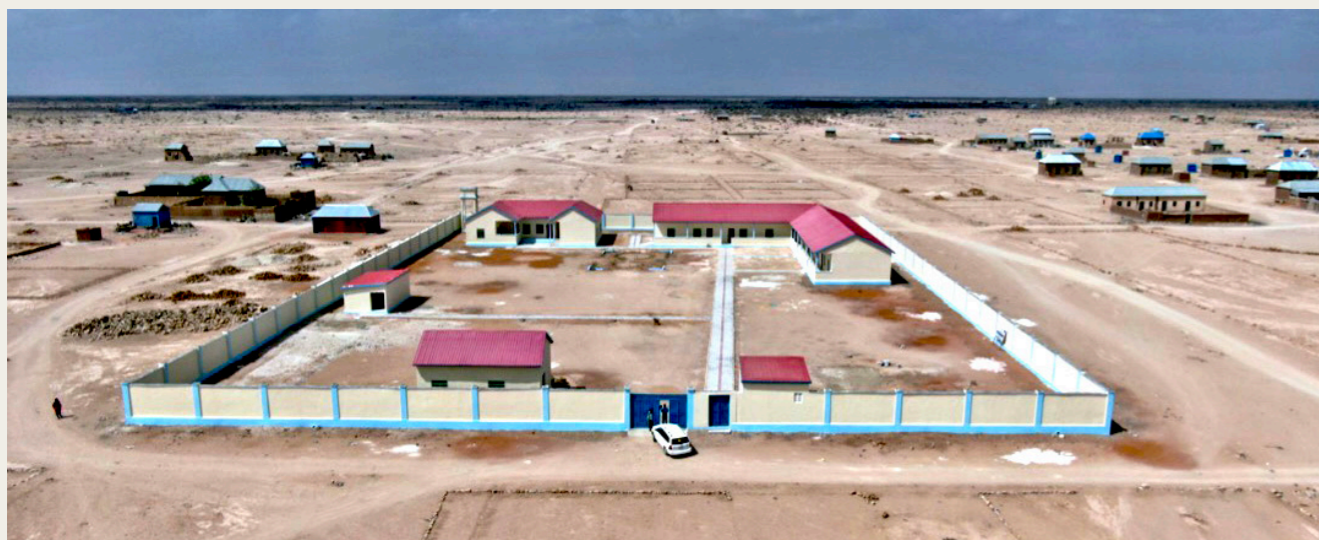
Photo: NIS. Construction of Adado school, Adado, Somalia
