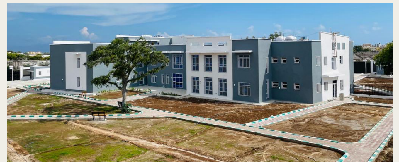
Photo: NIS. National Emergency Operations Centre, Mogadishu, Somalia.
