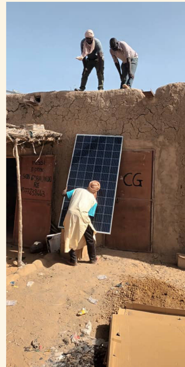
Photo: NIS. Home system installation, Forgho, Mali
