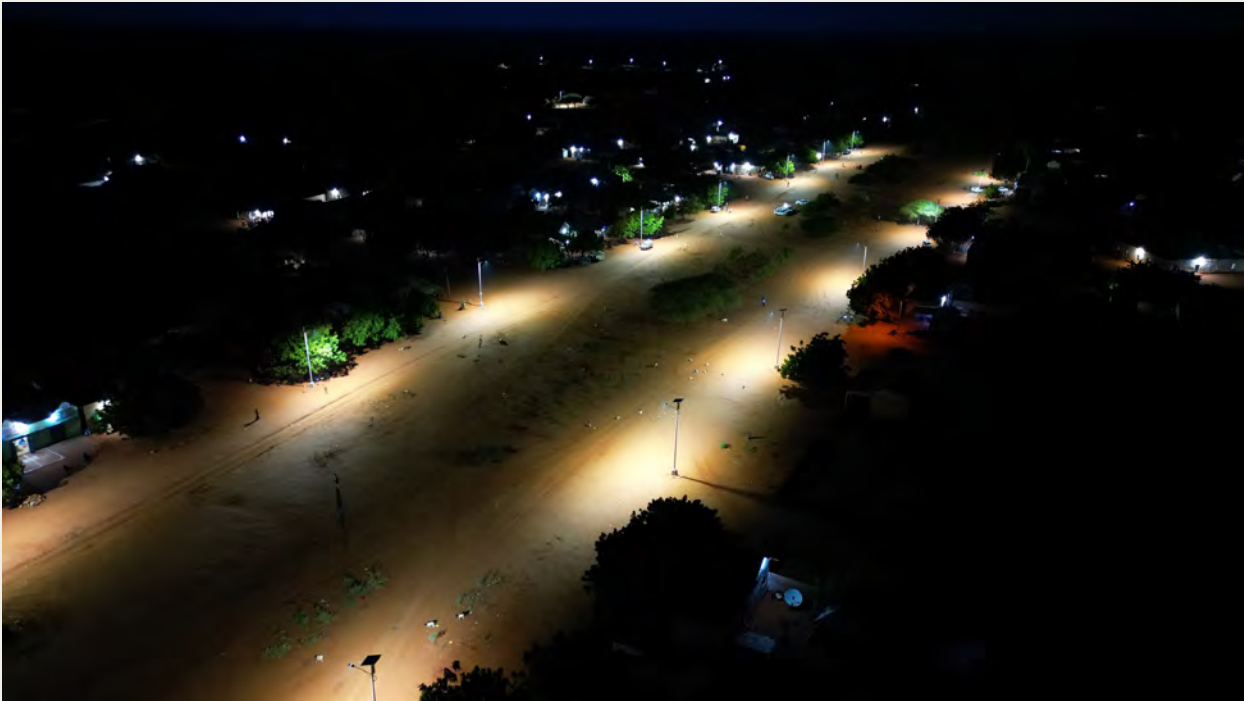
Photo: NIS. Solar Street Lights, Darussalam, Somaliab
